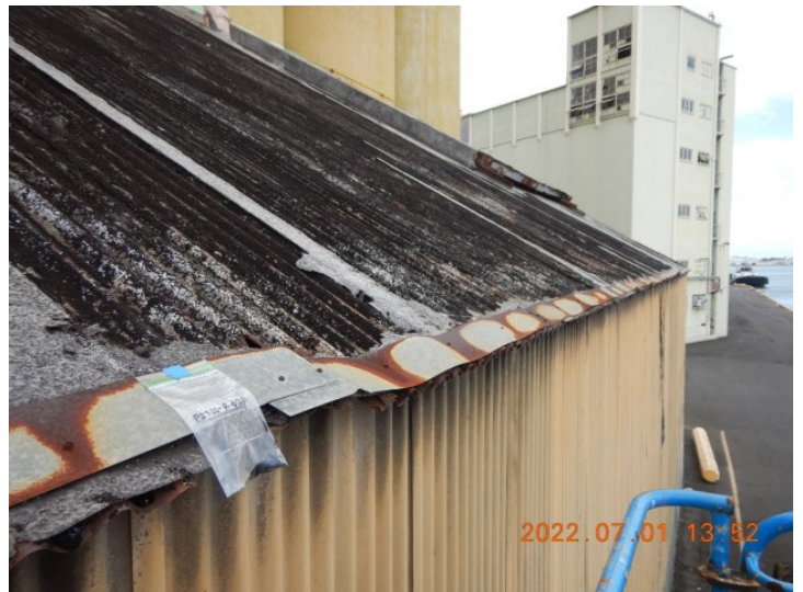
Photo 94 - P23SS-R-03B (Panoramic) [AL\DSCN7060.JPG]
