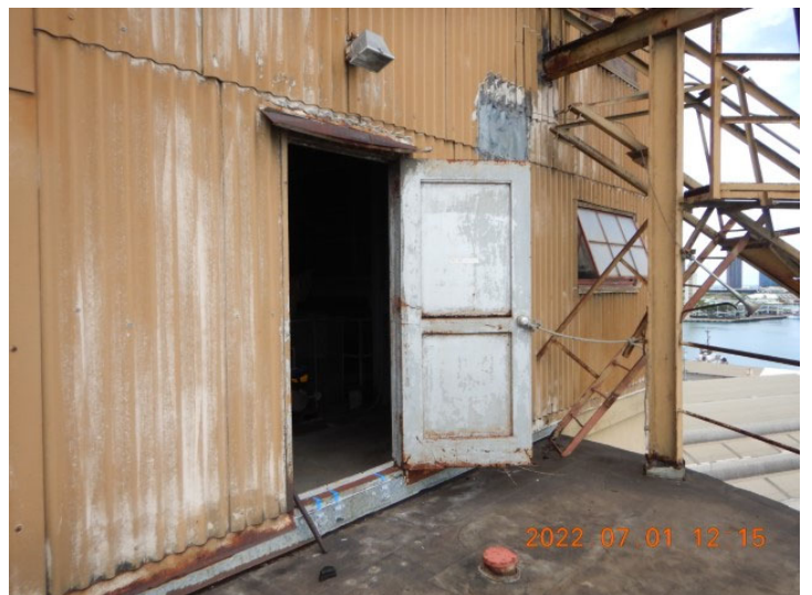
Photo 56 - P23SS-M-04C (Panoramic) [AL\DSCN6972.JPG]
