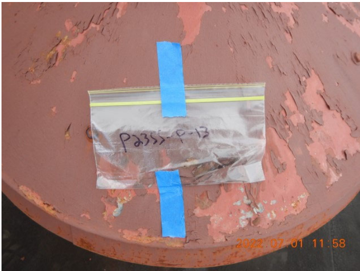
Photo 121 - P23SS-P13 (Close-up) [AL\DSCN6948.JPG]
