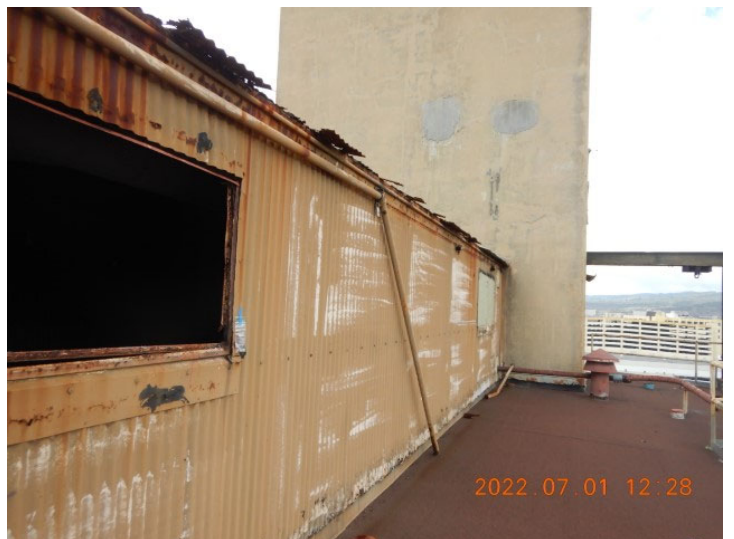
Photo 68 - P23SS-M-06C (Panoramic) [AL\DSCN6981.JPG]
