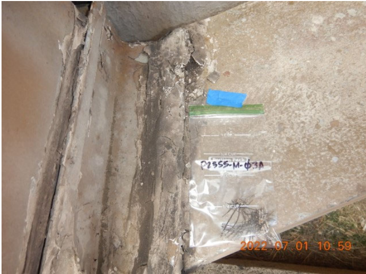
Photo 45 - P23SS-M-03A (Close-up) [BB\DSCN9196.JPG]
