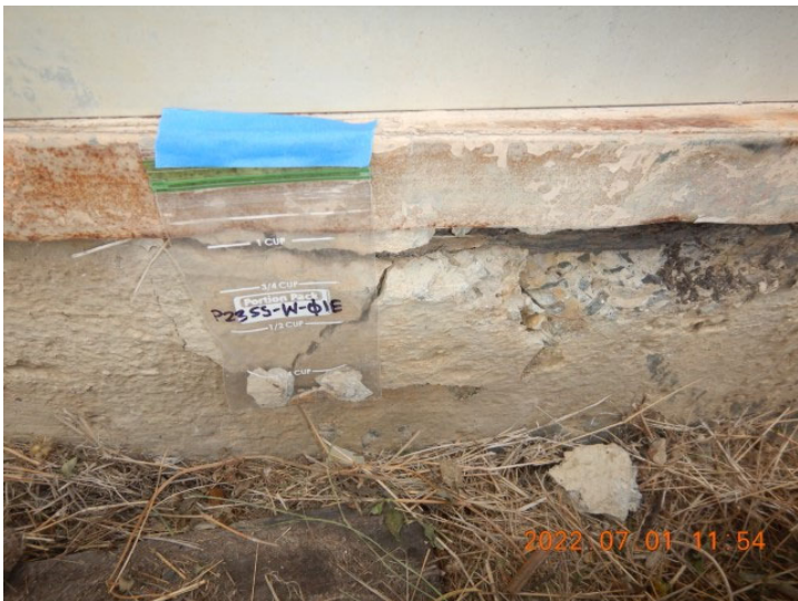
Photo 15 - P23SS-W-01E (Close-up) [BB\DSCN9227.JPG]
