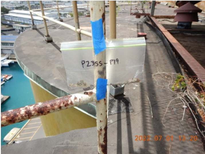
Photo 133 - P23SS-P19 (Close-up) [AL\DSCN7044.JPG]
