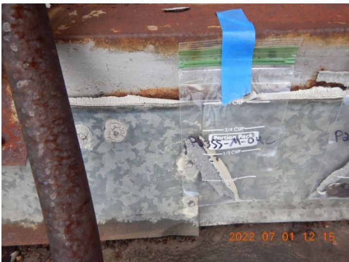
Photo 55 - P23SS-M-04C (Close-up) [AL\DSCN6971.JPG]
