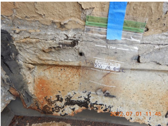
Photo 61 - P23SS-M-05C (Close-up) [AL\DSCN6946.JPG]
