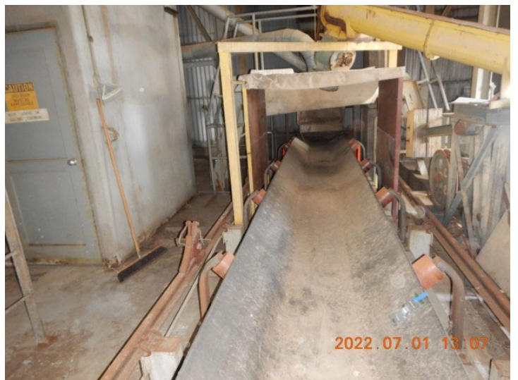
Photo 74 - P23SS-M-07C (Panoramic) [AL\DSCN7033.JPG]
