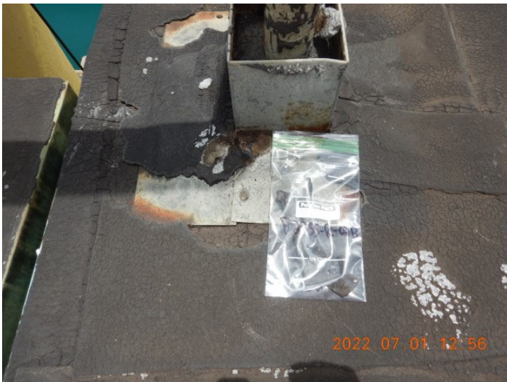
Photo 87 - P23SS-R-02B (Close-up) [BB\DSCN9244.JPG]
