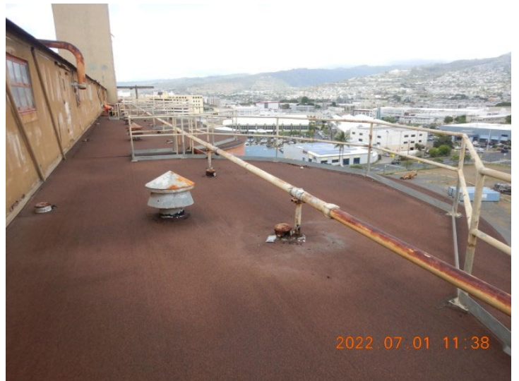
Photo 82 - P23SS-R-01B (Panoramic) [AL\DSCN6939.JPG]
