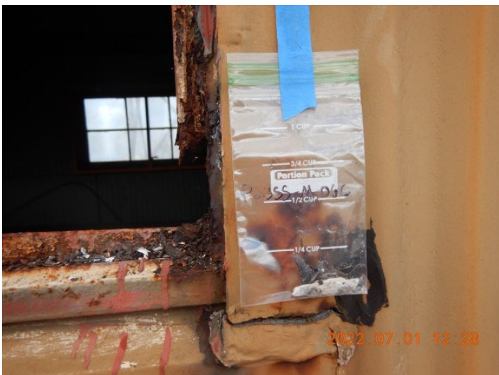
Photo 67 - P23SS-M-06C (Close-up) [AL\DSCN6979.JPG]
