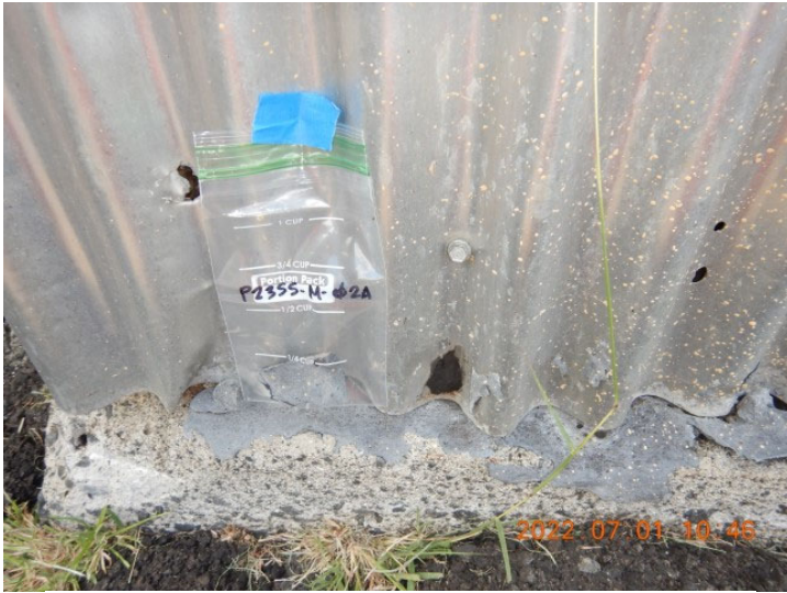
Photo 39 - P23SS-M-02A (Close-up) [BB\DSCN9188.JPG]
