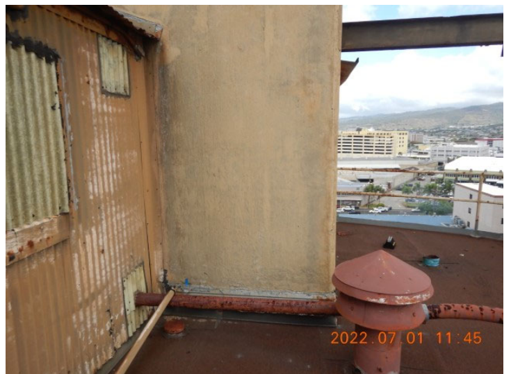
Photo 62 - P23SS-M-05C (Panoramic) [AL\DSCN6947.JPG]
